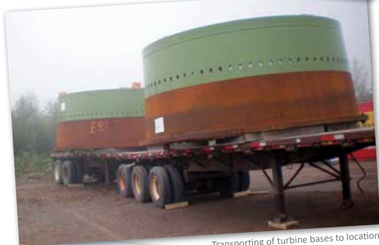
Turbine base being put in place for turbine 22
